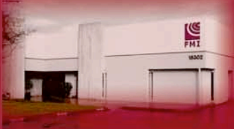
Huntington Beach, CA Facility
